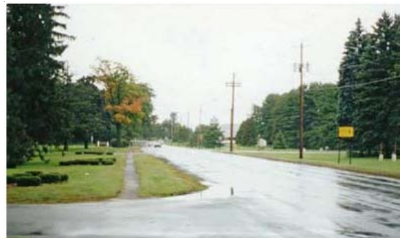
Figure 5a. Existing two-lane roadway
