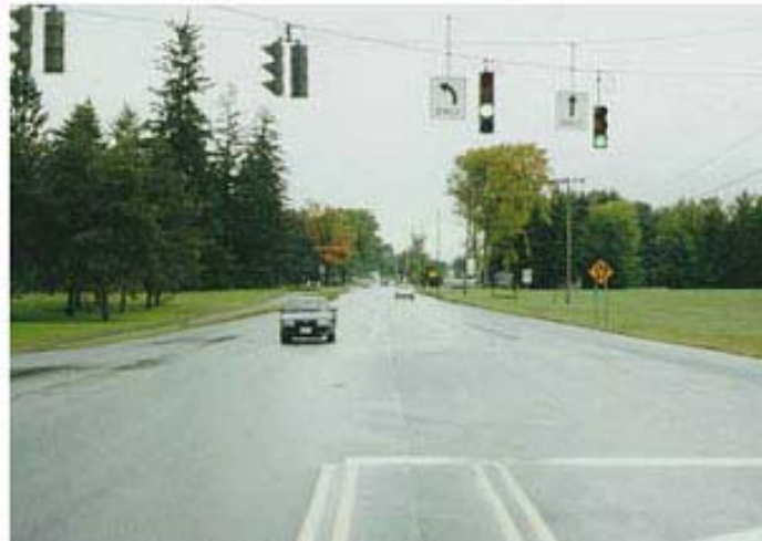
Figure 9a. Existing intersection
